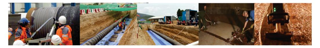
Defects repair on the existing pipeline with composite materials of various purposes, including repair of thru hole defects under pressure.
